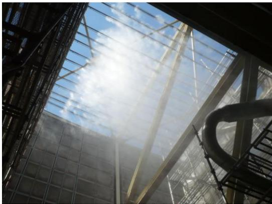
Photo 1. Nozzle array during spraying. Photo taken from below. Note scaffolds at left and right, and structural beams in center which capture some of the mist
